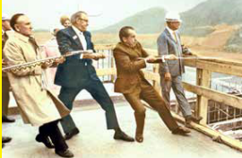
US President Richard Nixon helps with a ceremonial cement pour during construction of the Libby Dam, September 25, 1971.
